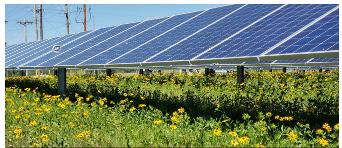
Selecting plant species that are able to tolerate some shading are an important consideration.
