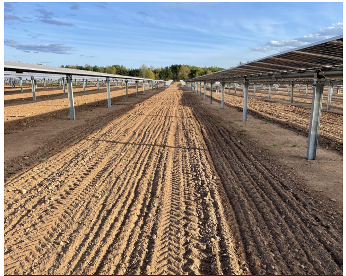
Properly completed and timed site preparation techniques are critical to the overall success or failure of the vegetative cover establishment on solar sites.
